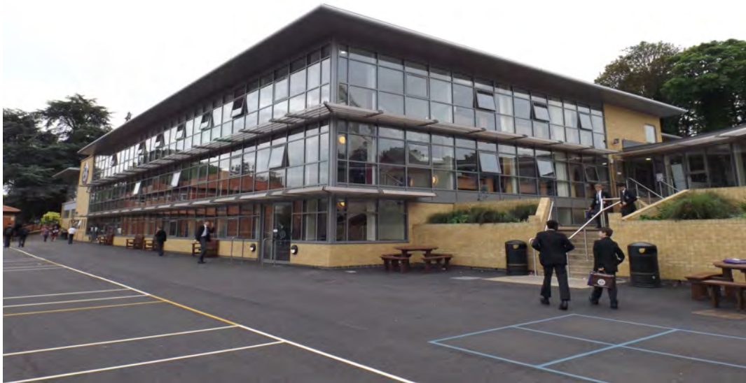
ST COLUMBA'S COLLEGE, King Harry Lane – Extensions to Gymnasium, New Foyer, etc.
